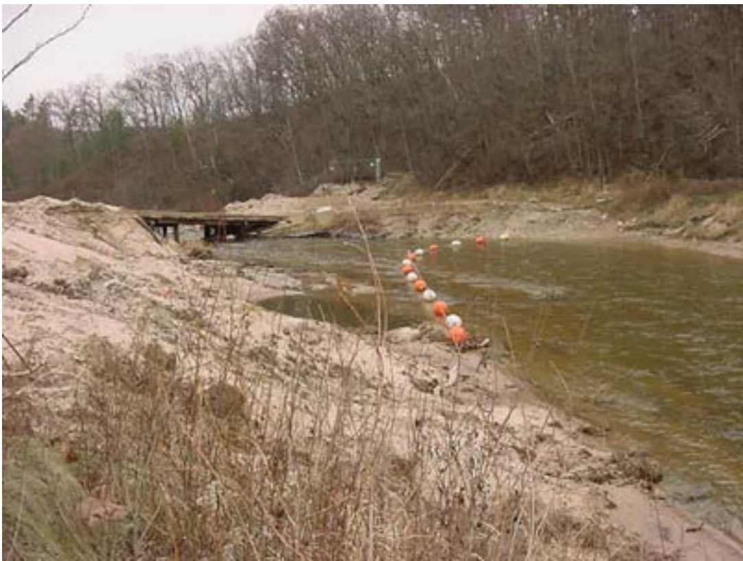
Removal of Stronach Dam near completion, November 2003, Stronach, Michigan
