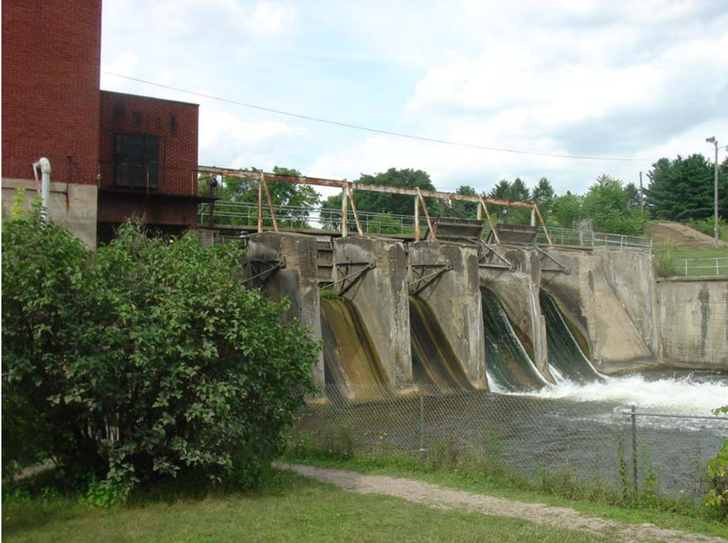
Pucker Street Dam, Niles, Michigan
