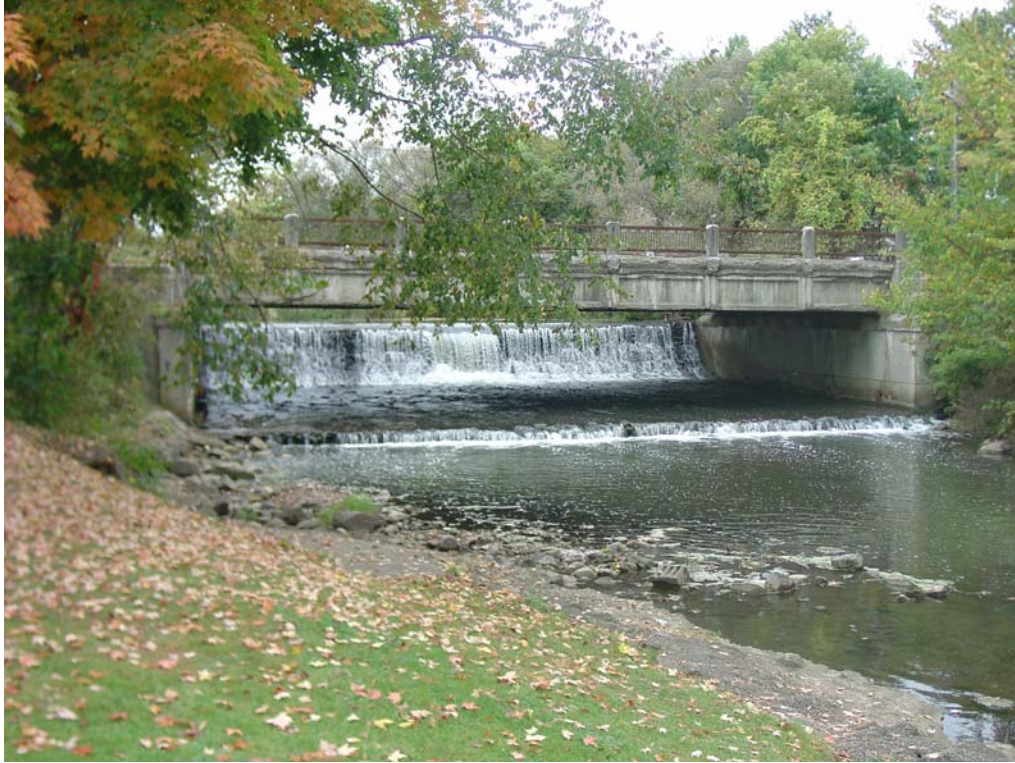
Mill Creek Dam, Dexter, Michigan
