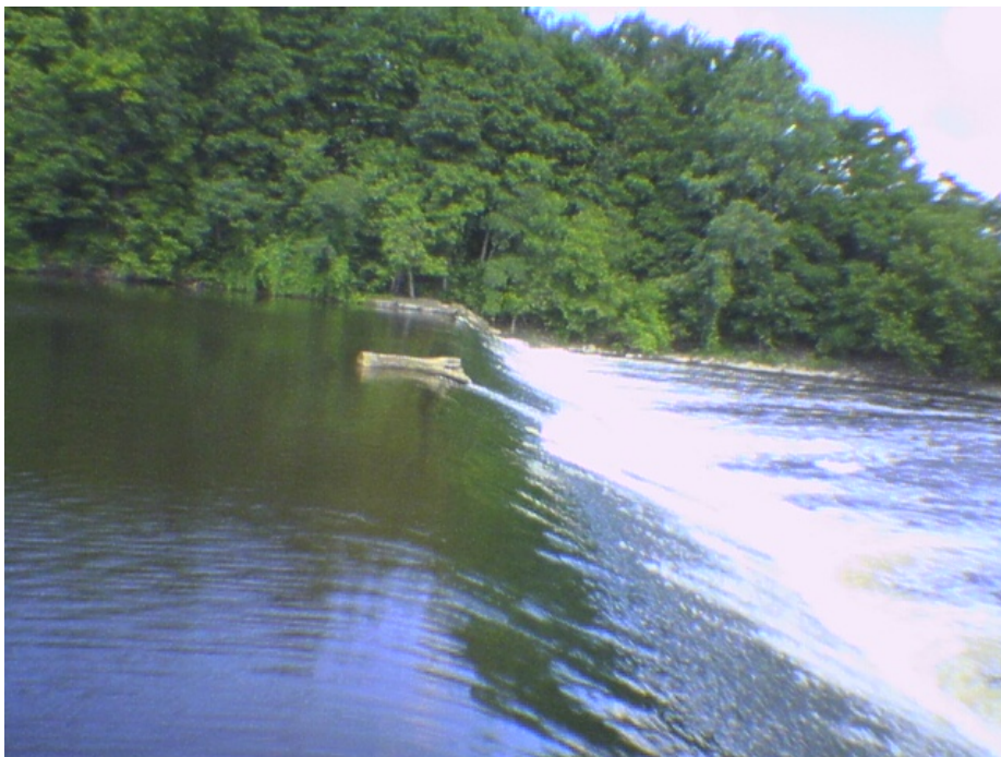
Lyons Dam, Lyons, Michigan
